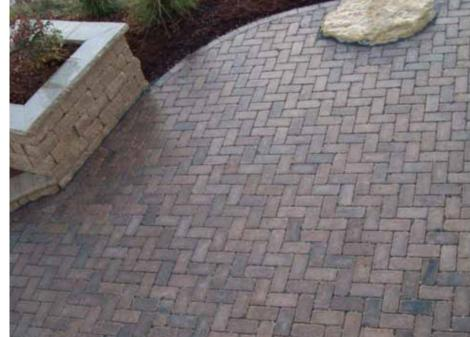
Eco-Priora<sup>™</sup> is a simple rectilinear shape that comes with several surface textures and is designed with special spacer bars located along the sides of each stone unit. The resulting 7 mm gap is filled with a clear fine stone chip that allows the rapid penetration of rain water into the sub-base and subsoil.
