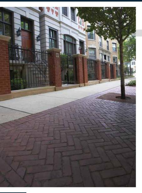
With Copthorne® you can create a street paver look reminiscent of the brick pavers used in old European cities, towns and villages. Crafted using a special forming process, each piece is uniquely altered, yet the dimensions are consistent for easy, efficient installation. The result is a realistic look with the long-lasting durability of concrete.
